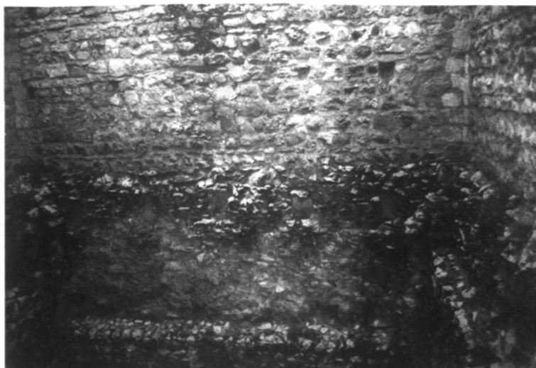
St Leonard's Tower: removed masonry at the internal offset level (south and west walls). Photograph: author
