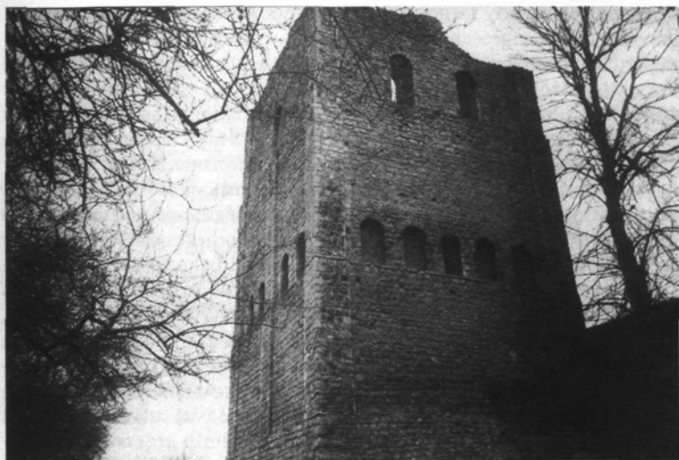
St Leonard's Tower: blind recesses in the south and east faces.
