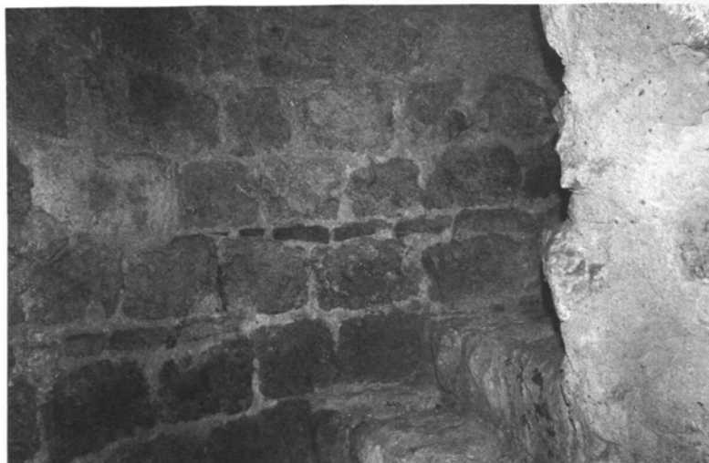
St Leonard's Tower: typical levelling courses in the vice wall. Photograph: author
